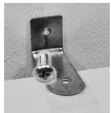
marked spot and insert a plug. Now hang the heater in place and screw the bracket to the wall, as shown in the diagram. The heater is now installed.
